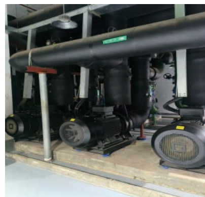
Replacement of Level 3 energy efficiency motors
