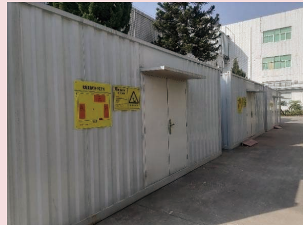
Hazardous Waste Temporary Storage Area
